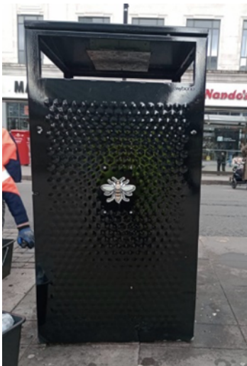
Image showing litter bin after the anti-graffiti coating is applied
